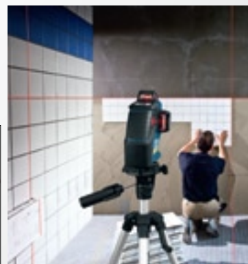
Level and Square to Install Tile
